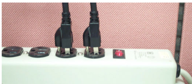
Figure 3.7: Power cord plugs should have same orientation in the socket/ 插座上电源线方向相同 / 插座上的電源線方向應相同
