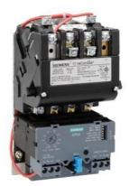
Non-reversing motor starter Size 0 Single phase full voltage Solid-state overload relay OLRelay amp range 5.5-22A 24VAC 50-60HZ coil Combination type No enclosure
