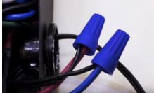
**6** Connect transformer to low voltage LED wiring using wire nuts: red (+) positive, blue negative (-) Note: If using Inspired LED interconnect cables, cut off one end connector, split and
