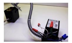
Using in-wall rated or armored cable, run wires from compatible wall switch through wall box or directly to location of transformer
